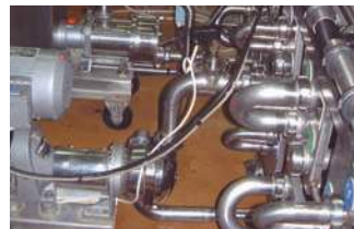
S4C FOR CONDITIONING
